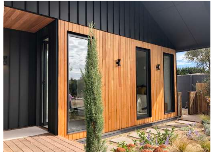
Architect: S. Group Official
